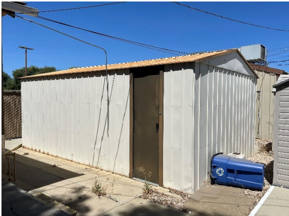
-109 West E Street – Metal Building-
