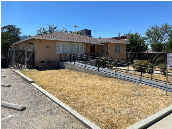
-116 West F Street - Exterior-
