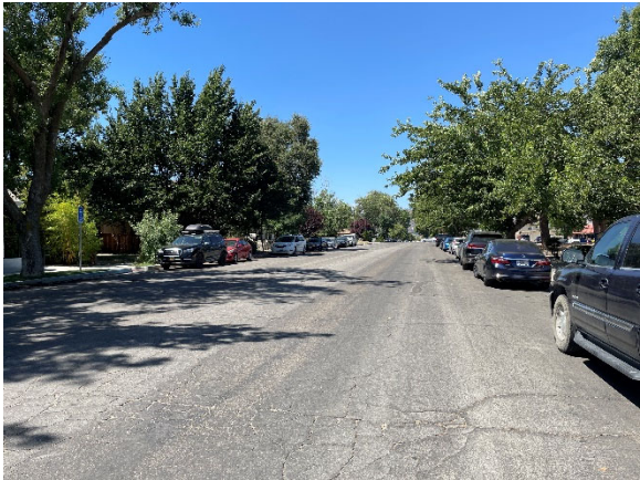
-West E Street Facing West-
