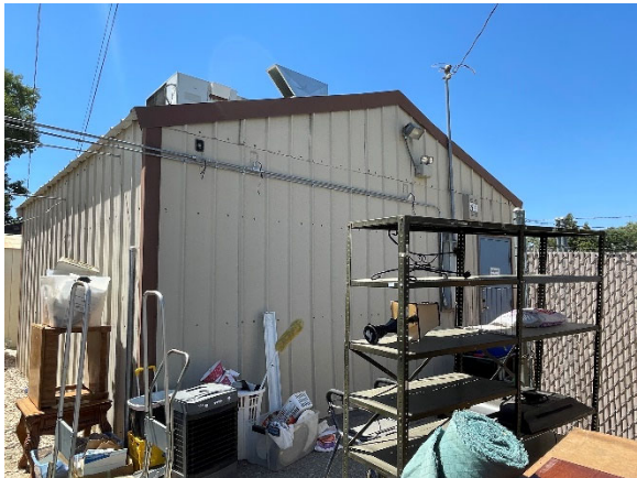
-109 West E Street – Metal Building-
