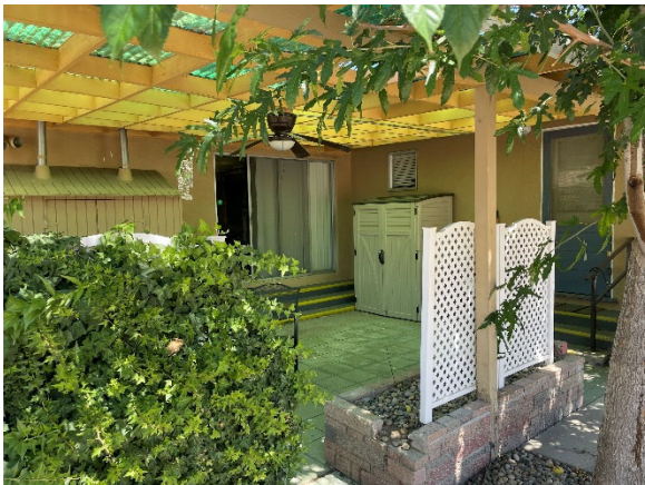
-116 West F Street - Exterior-
