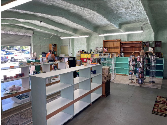
-101 West E Street – Metal Building Interior-
