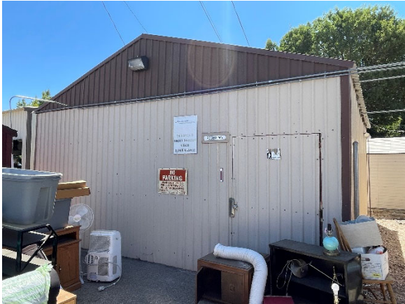
-109 West E Street – Metal Building-
