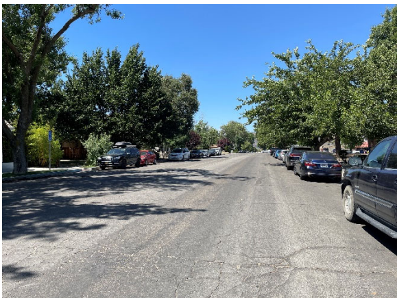
-West E Street Facing West-
