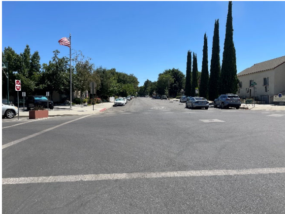
-West E Street Facing East-
