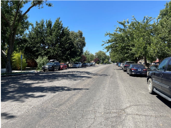
-West E Street Facing West-
