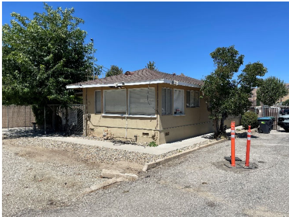
-116 West F Street - Exterior-
